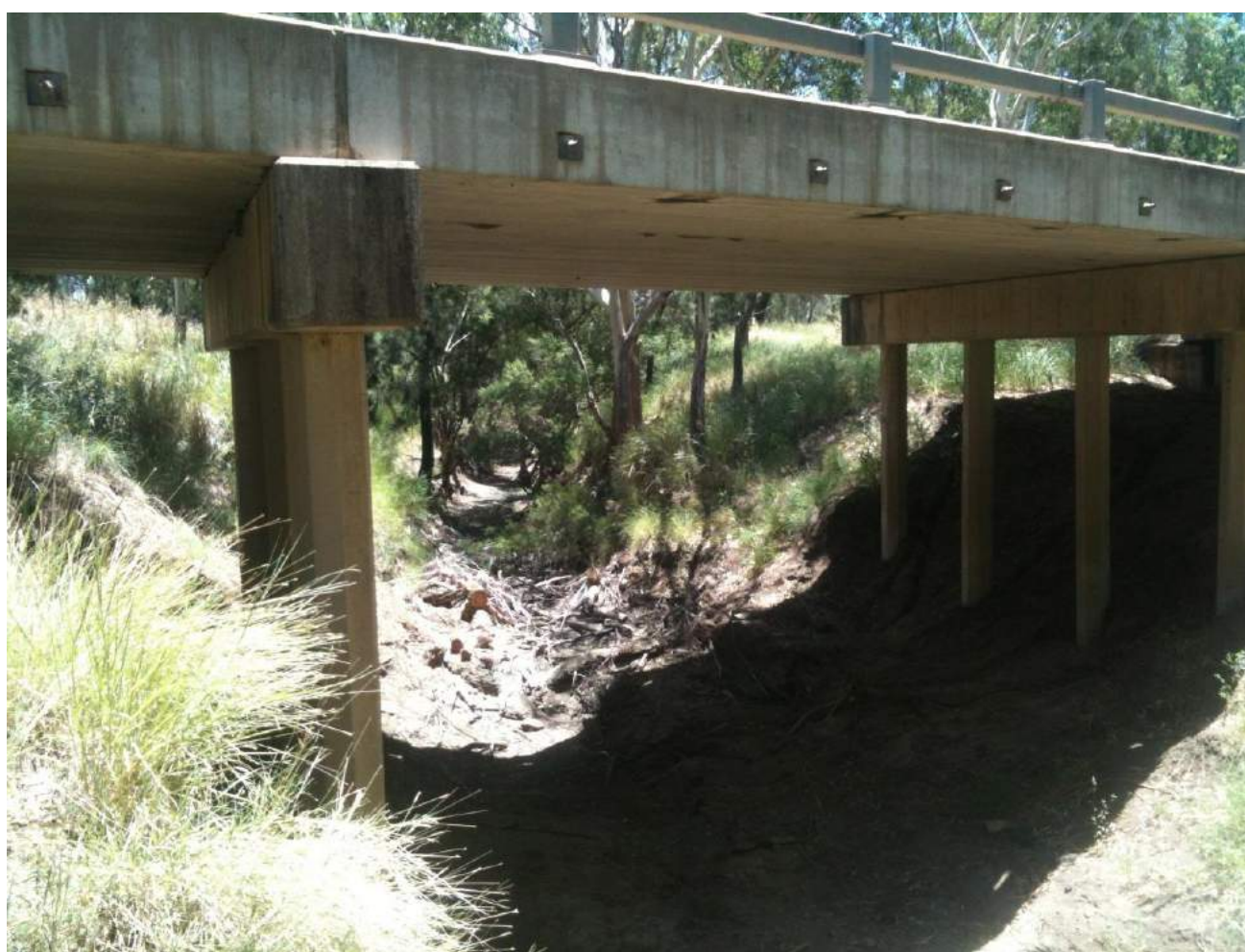
Plate 2: Aldebaran Creek channel at the Dawson Highway
